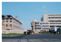
TBR Plant in Xiasha
